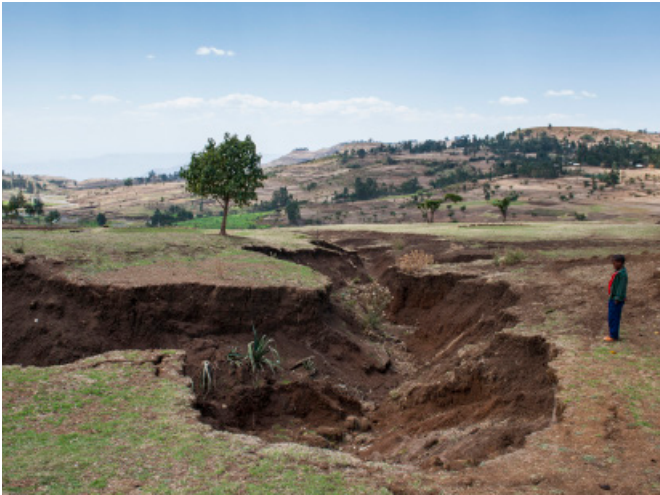
Before: erosion ditches
