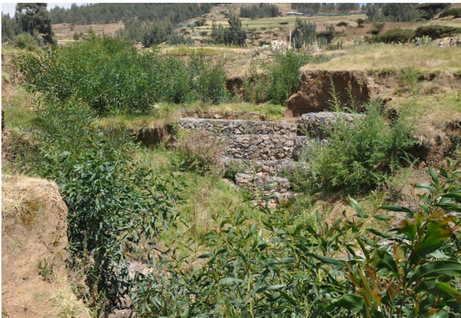
Wire baskets filled with stones are strategically placed within the ditches.
